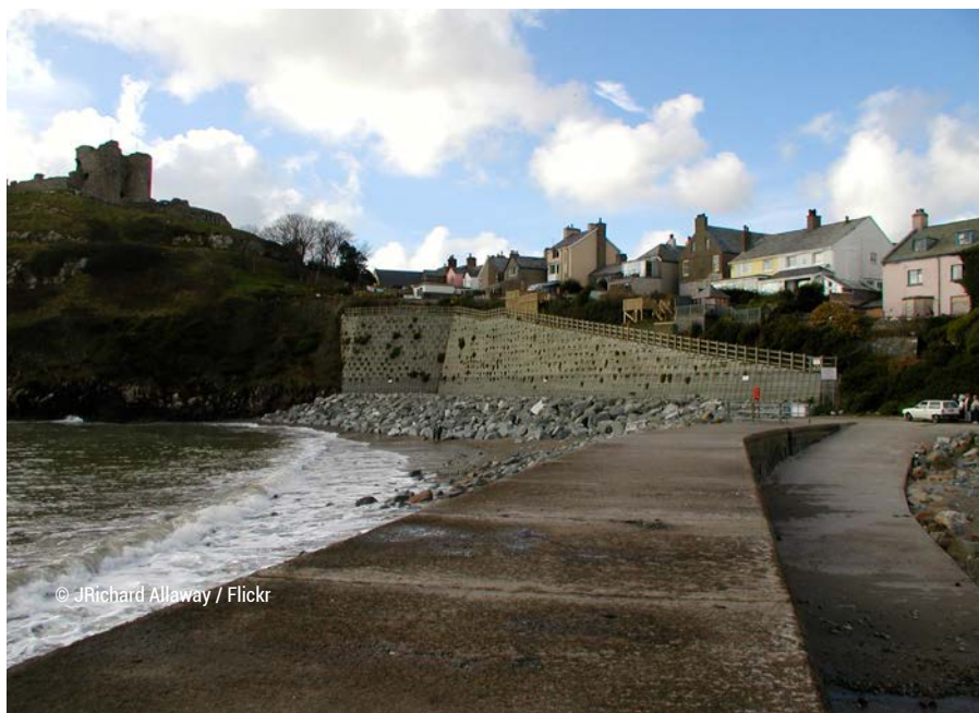
Figure 12: Coastal erosion management, Criccieth, North Wales, UK
